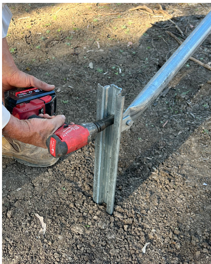
Ratchet drive M8 bolt to attach OKWAS/B8 bracket to angle stay
