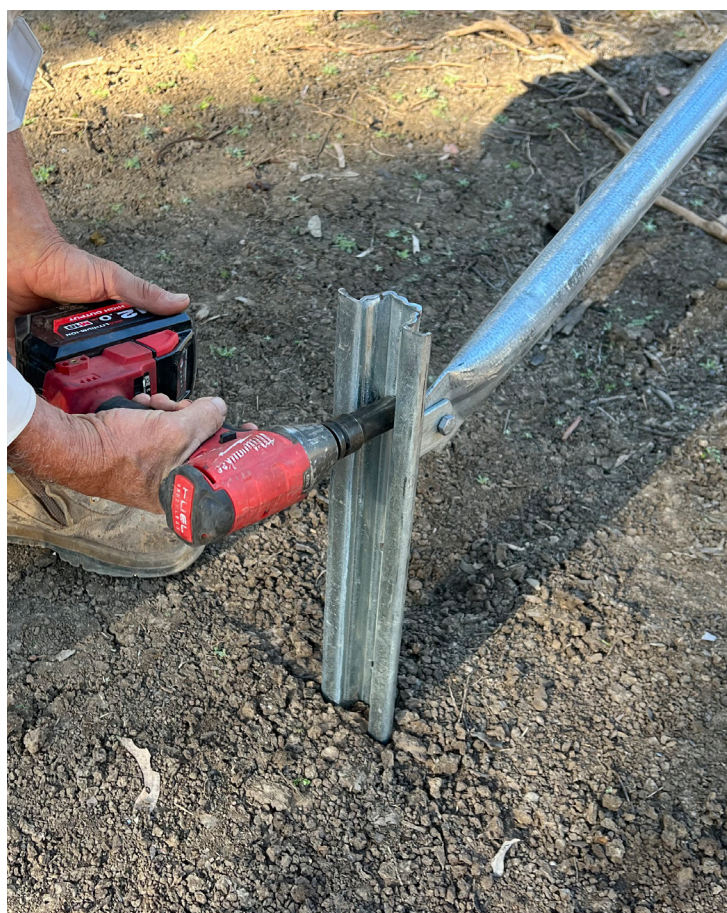
Ratchet drive M8 bolt to attach OKWAS/B8 bracket to angle stay
